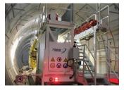
A perfect fit – the first drilling rig drills all the holes that will accommodate brackets for cabling, walkways and fire mains. The second machine focusses on the holes for the overhead electricity line, which will power the Crossrail trains.
