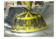
Crossrail drilling rig working in the Thames Tunnel, which stretches for almost two miles beneath the city of London. Eaton's Heavy Duty Series of axial piston pumps supply the hydraulic oil for the hydraulic systems that manipulate the arms and control the 36 drills.
